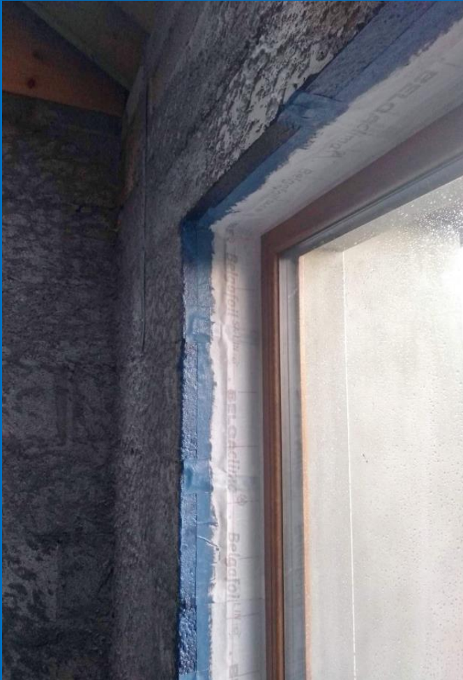
Correct tape used and sealed with airtightness paint
