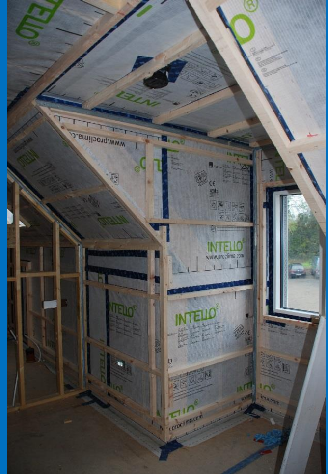
Well sealed membrane to dormer roof
