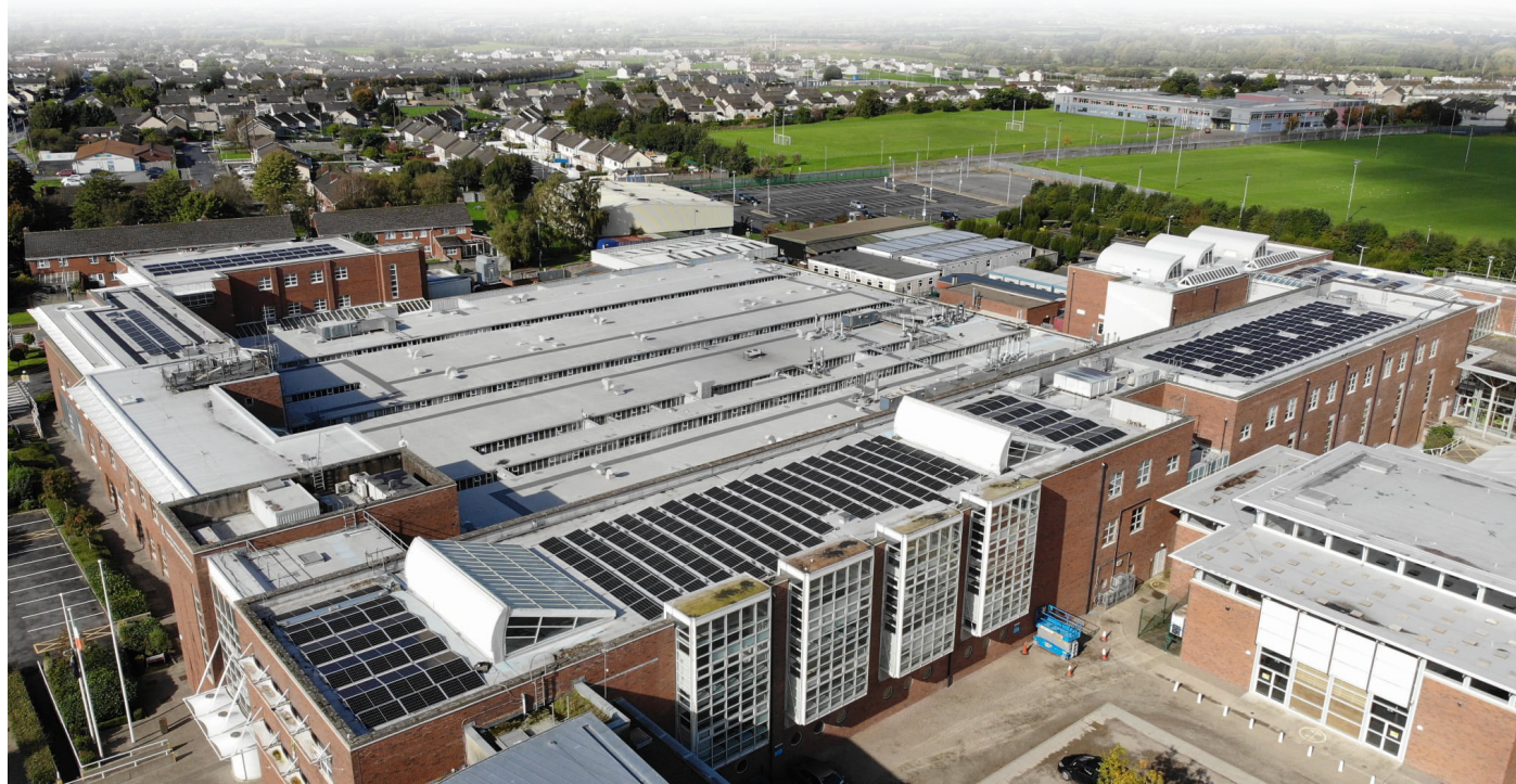
166 kWp of a solar photovoltaic (PV) system on the main building of the Technological University of the Shannon
